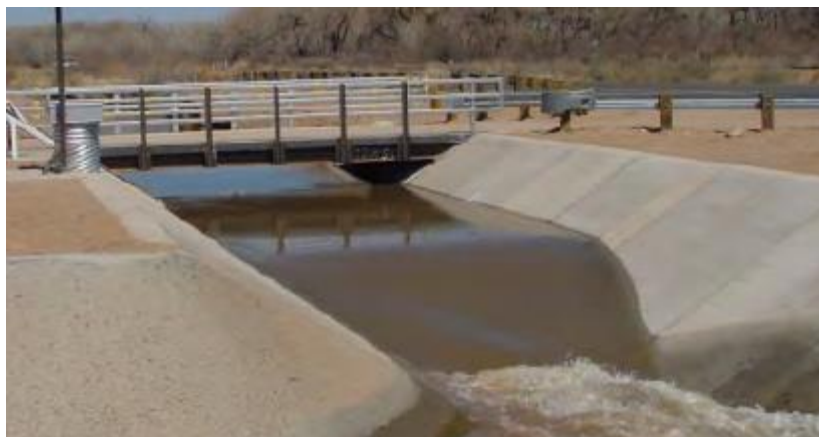
Fig. 1. Example of the broad crested weir
